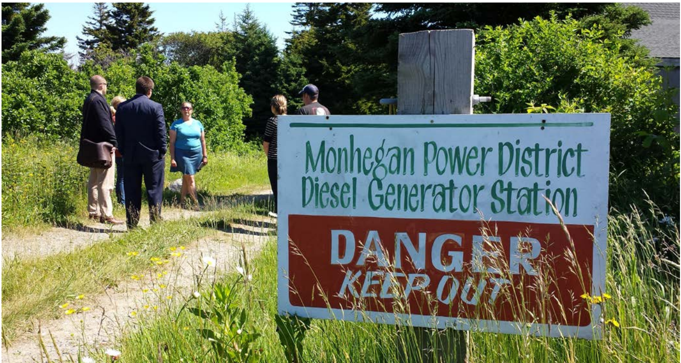
Monhegan Island residents brief state leaders on local energy challenges, including the high cost of diesel-generated power.
